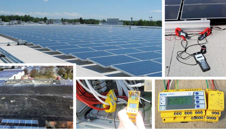
importance that the photovoltaic system is permanently monitored in order to display the occurrence of residual currents as early as possible so that the problem can be solved as soon as possible.
