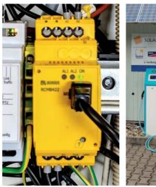
Figure 7: RCMB 420 EC 1 channel
