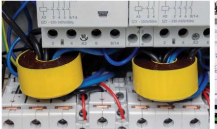
Figure 6: RCMB 420 EC 2 channels
