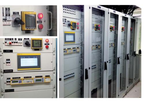
lation fault location in group two rooms by Bender, residual current monitoring for TN-Systems by Bender, power quality analysers by Bender and Condition Monitor CP700. All devices are integrated in the CP700 touch control panel for convenient system handling and overview.
